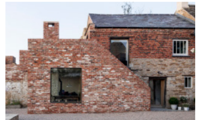
Figure 47: Recycled and reclaimed bricks used for an extension to a traditional dwelling in Gretton, UK.
