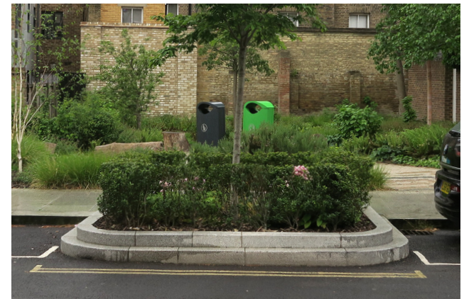
Figure 43: Kerb build out with street greening and SuDS installation, double kerb to prevent vehicle overrun.
