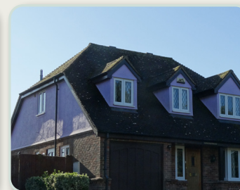
Clay tile clipped gabled roof with dormers
