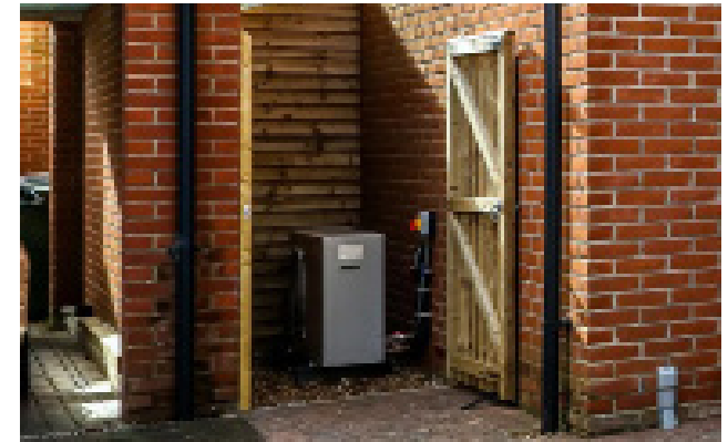
Figure 46: Example of a visually screened heating pump appropriate to the context of the building vernacular.
