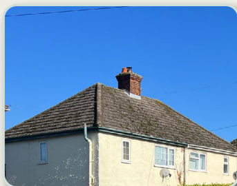
Brown clay tile hipped roof with chimney stack
